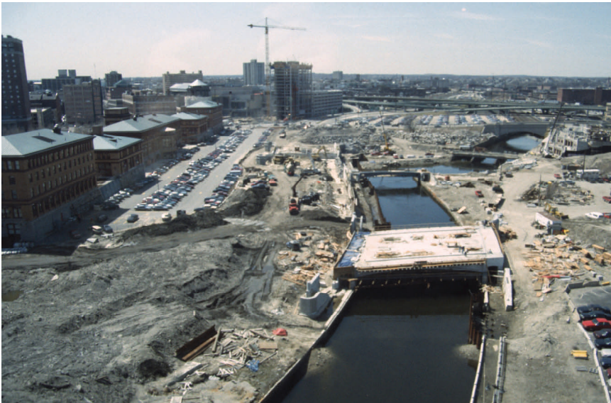
Moving the river through the Capitol Center, Providence, RI
